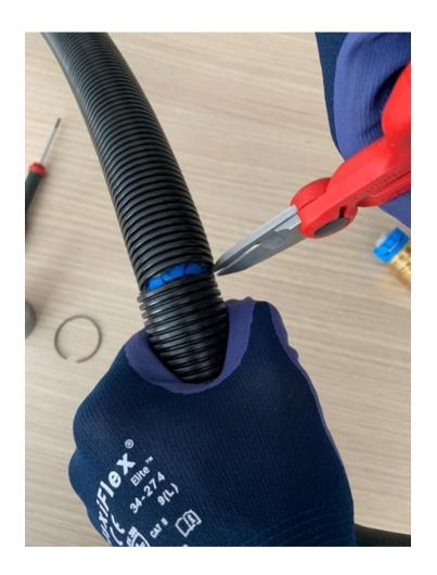
Cut the outer corrugated hose at the desired point or length
